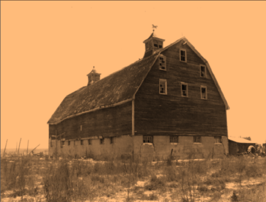
Figure 56 Shields Barn, NW 18-9-19W, 1910-12: southeast view.
