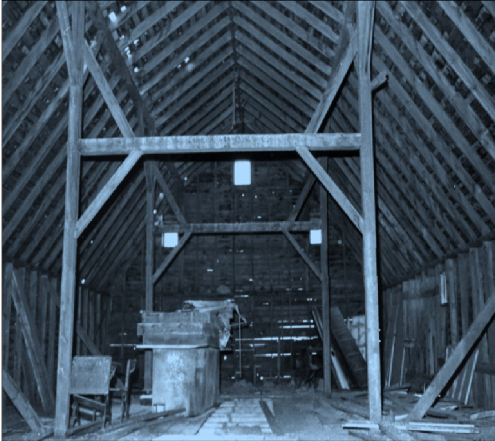
Figure 54 Roddick Barn. The builders of Nova Scotia style barns concentrated the main structural supports away from the walls, increasing internal stability and freeing the external walls for frame construction.
