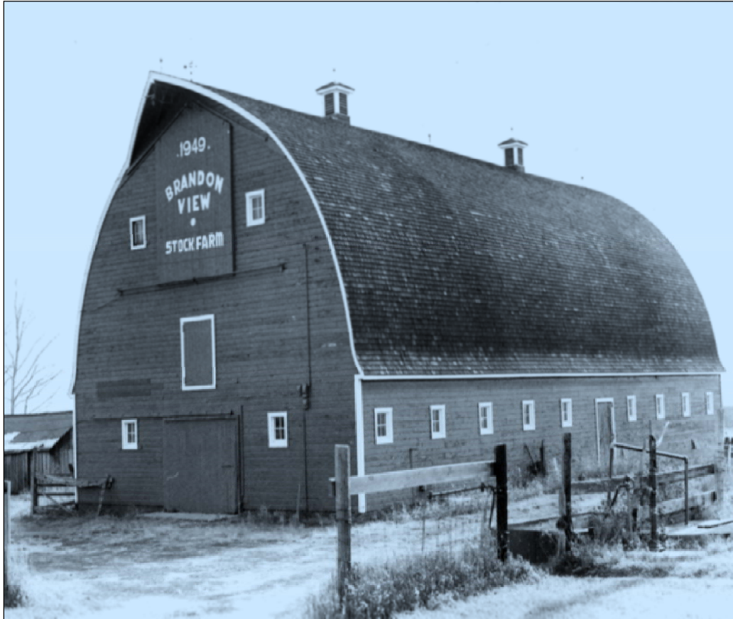
Figure 60 Hamilton Barn, NW 34-10-19W, 1949. The roof of this barn was constructed with laminated trusses that were built in Souris.
